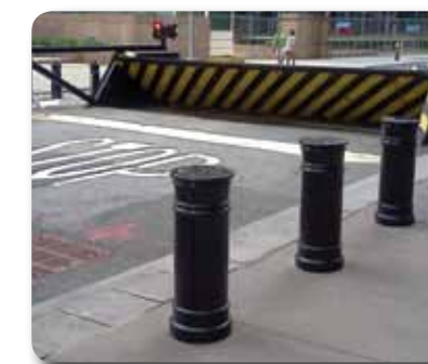
▶ Wedge and bollard control
